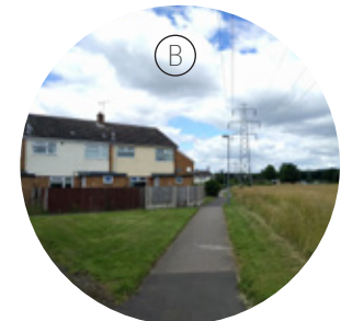
Pylons line the eastern edge of the Hallam Road Estate
